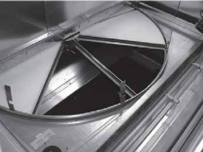
Figure 107. Segment Removal
